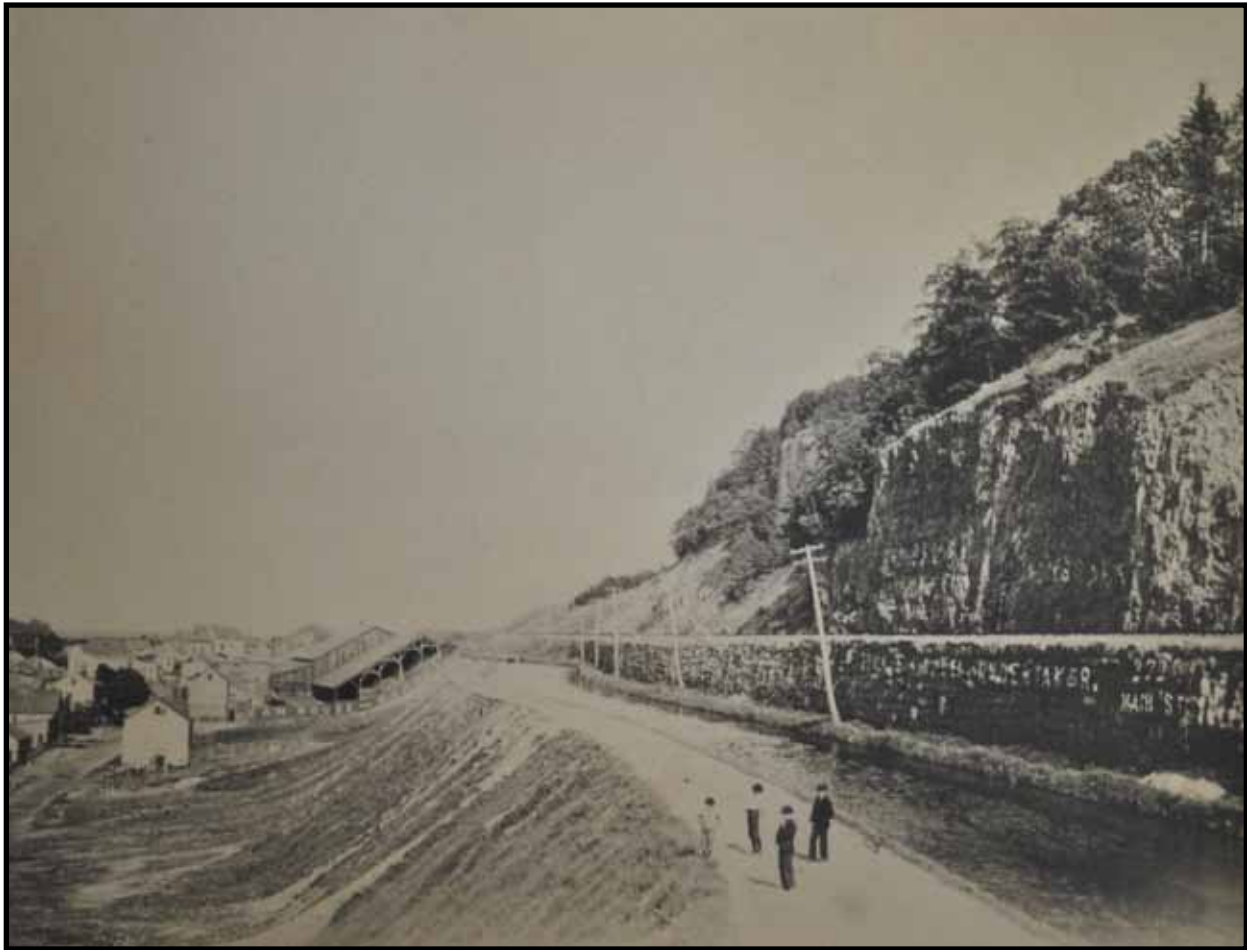
Photograph 2.2. View looking east on Grand Street toward the Dublin neighborhood with the Morris Canal at right. Circa 1880. Source: Passaic County Historical Society.
