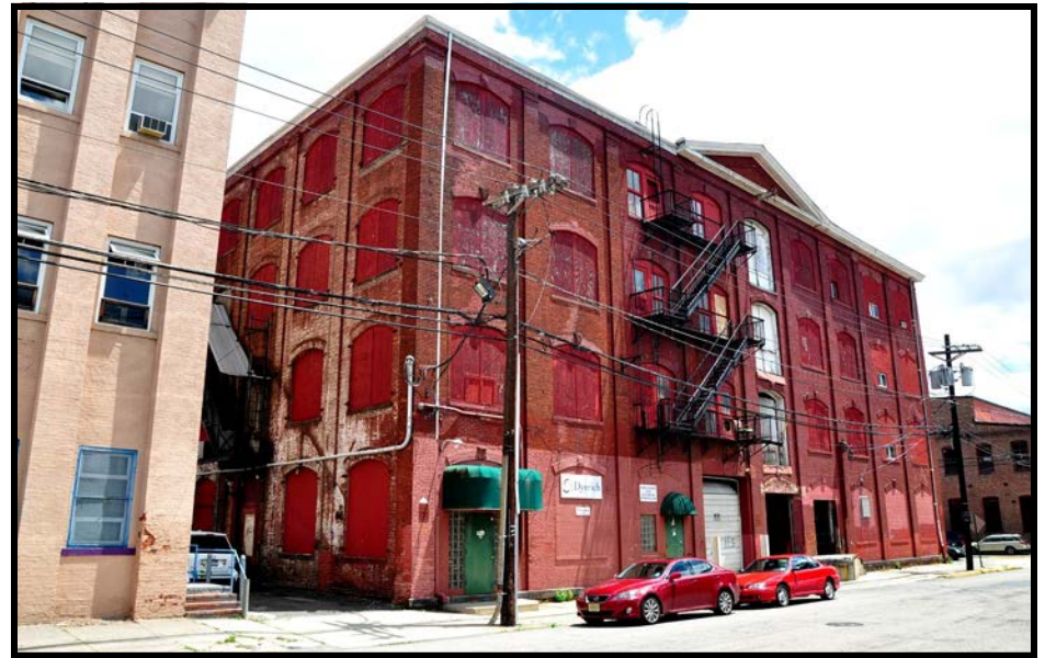
BARNERT 4: oblique overview of N and W sides, looking SE from Dale Ave. Note additions of loading docks and converted entrances at center of W side.
