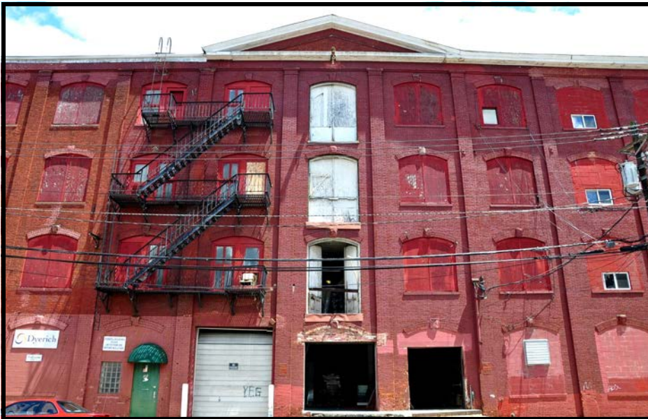
BARNERT 3: detail view of W side, looking E from Dale Ave. Note central hoisting bay over four converted entrances.
